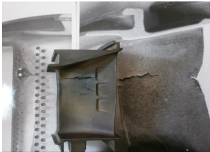
Figure 1. Localization of HPT nozzle blades damages in a zone of maximum temperatures action (in 1...2 mm spots).
